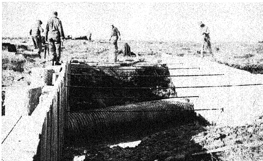
Figure 44. Corrugated metal culvert (thirty-six inch diameter) being con- structed within wooden bulkheads, before being filled with earth
